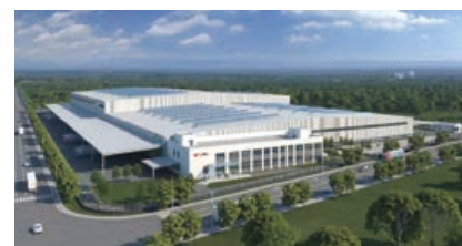
Xiaohudao Guangzhou Smart Factory
