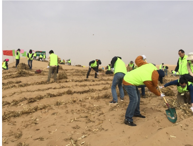
Straw checkerboard barriers were established before tree planting
