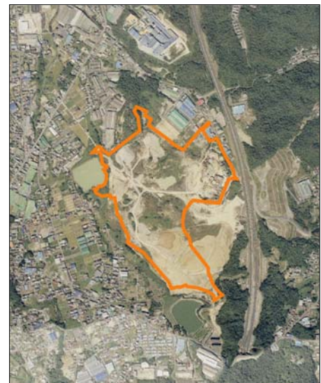
Planned construction site
