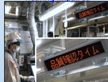
Electronic signage installation
